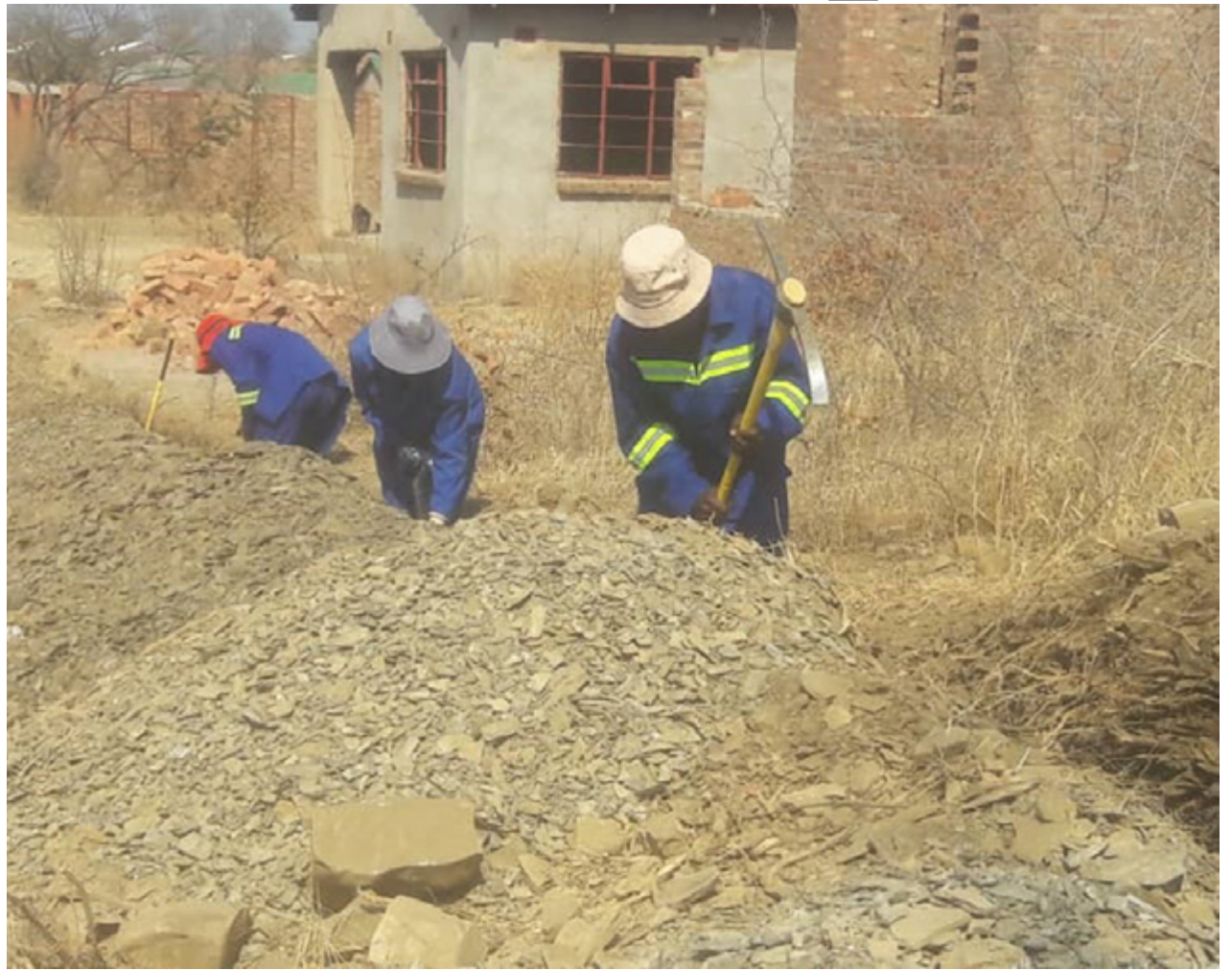
Digging trenches for laying of water pipes
