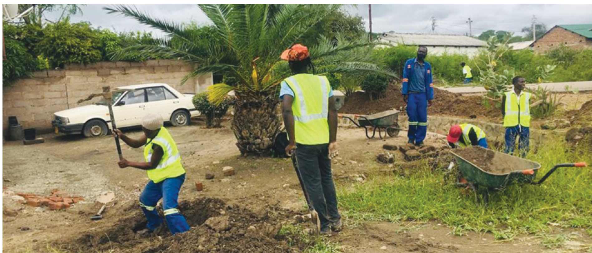
HLB workers digging trenches in Empumalanga suburb
