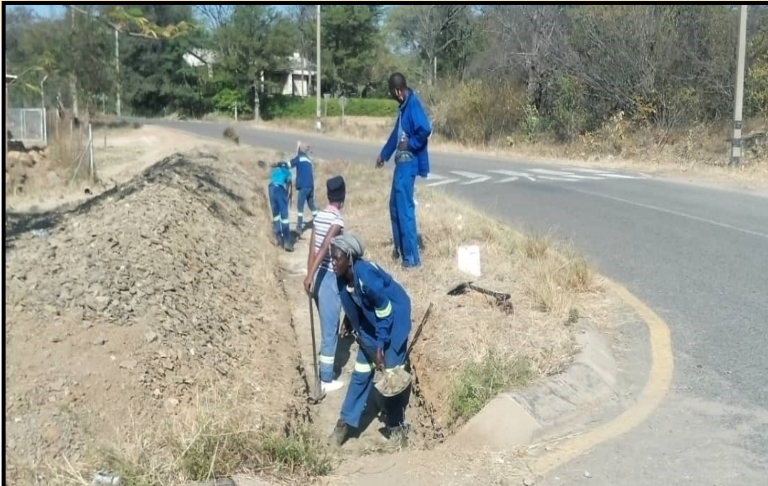
Hwange Local Board employees clearing a storm water drain
