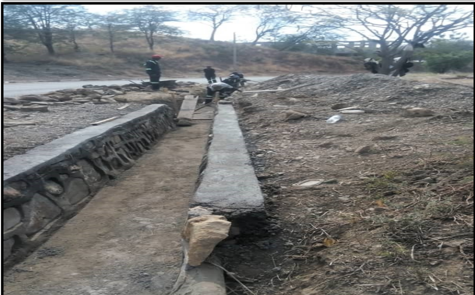
Hwange Local Board employees embarking on storm water drainage stone pitching
